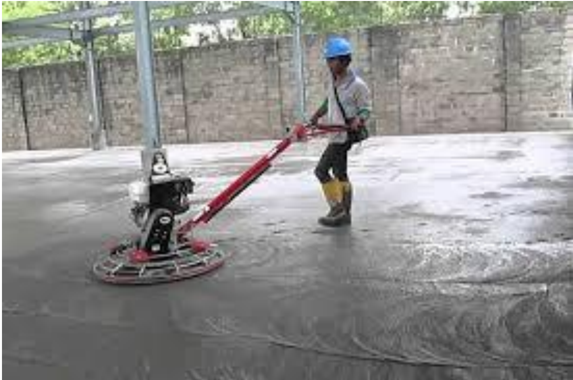
Fig 2.1.1. Process of Tremix floor
