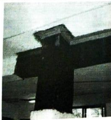
Fig. 6.1.4(e) : FRP jacketing for rectangular RCC column used in RCC structural rehabilitation
