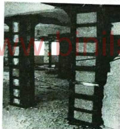
Fig. 6.1.4(d) : Shows steel jacketing for rectangular RCC column used in RCC structural rehabilitation
