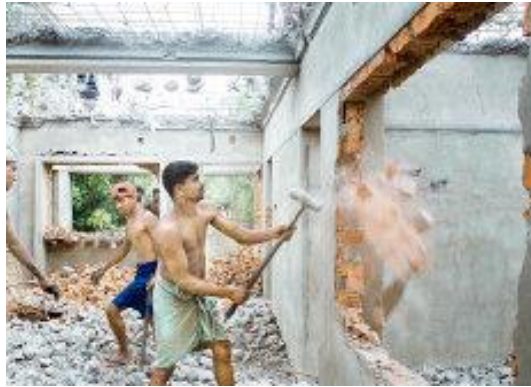
Figure : Demolition By Hand
