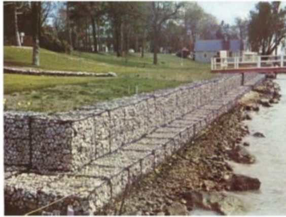
Bulkhead structure constructed by Gabion mesh boxes
