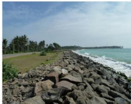
Figure Rubble mound seawall protecting the coastal road at Madampagama, SW coast of Sri Lanka.
