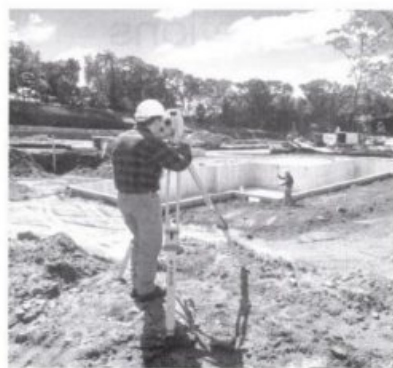
Measuring with a total station
