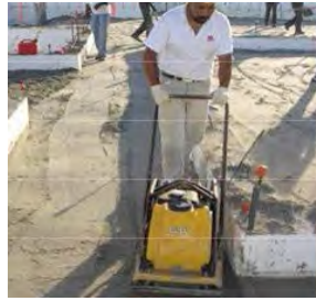
2.2.2.5(i) Surface Vibrator
