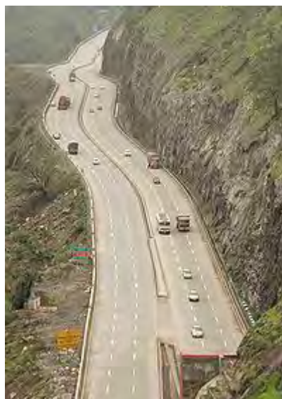
1.4.11 (a) Mumbai-Pune Expressway
