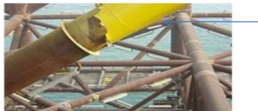
Fig. 2.2.4 Aluminium Sacrificial anode
